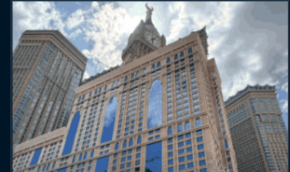
Al Safwah Tower 3
